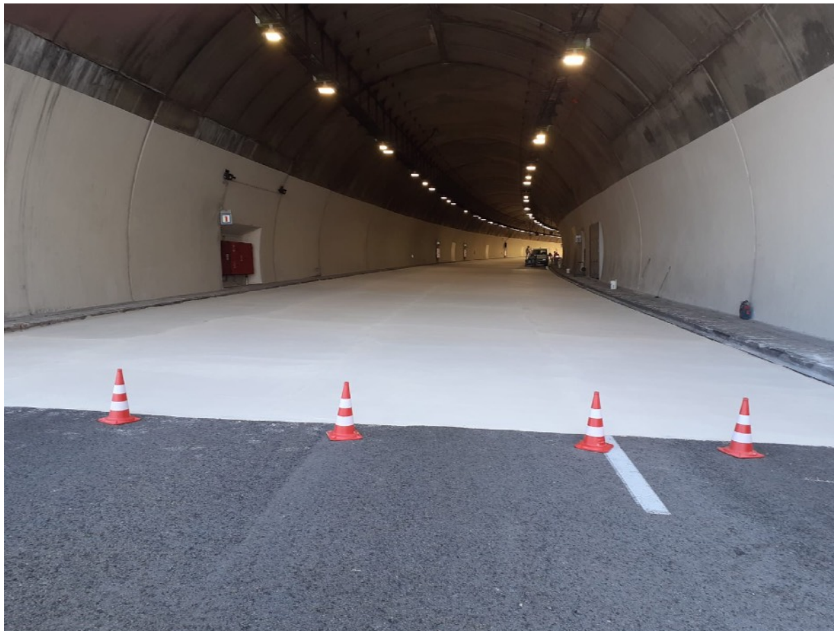
Olympia Odos – Tunnel Teseo
